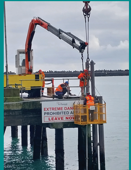
The stainless steel pole that houses the tsunami monitoring equipment is lifted and placed in the water and secured to Blyde Wharf.
